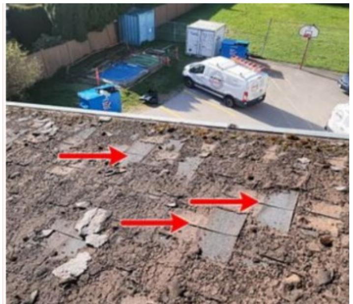
**Worn out roof shingles are causing a roof leak**
